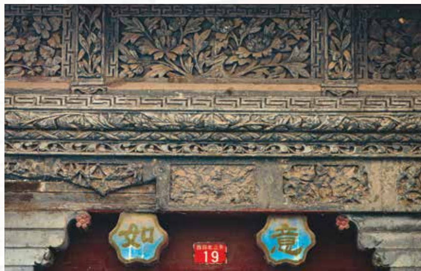
▼ Brick-carved decorations on the main gate lintel of a courtyard in Xisibei Santiao
